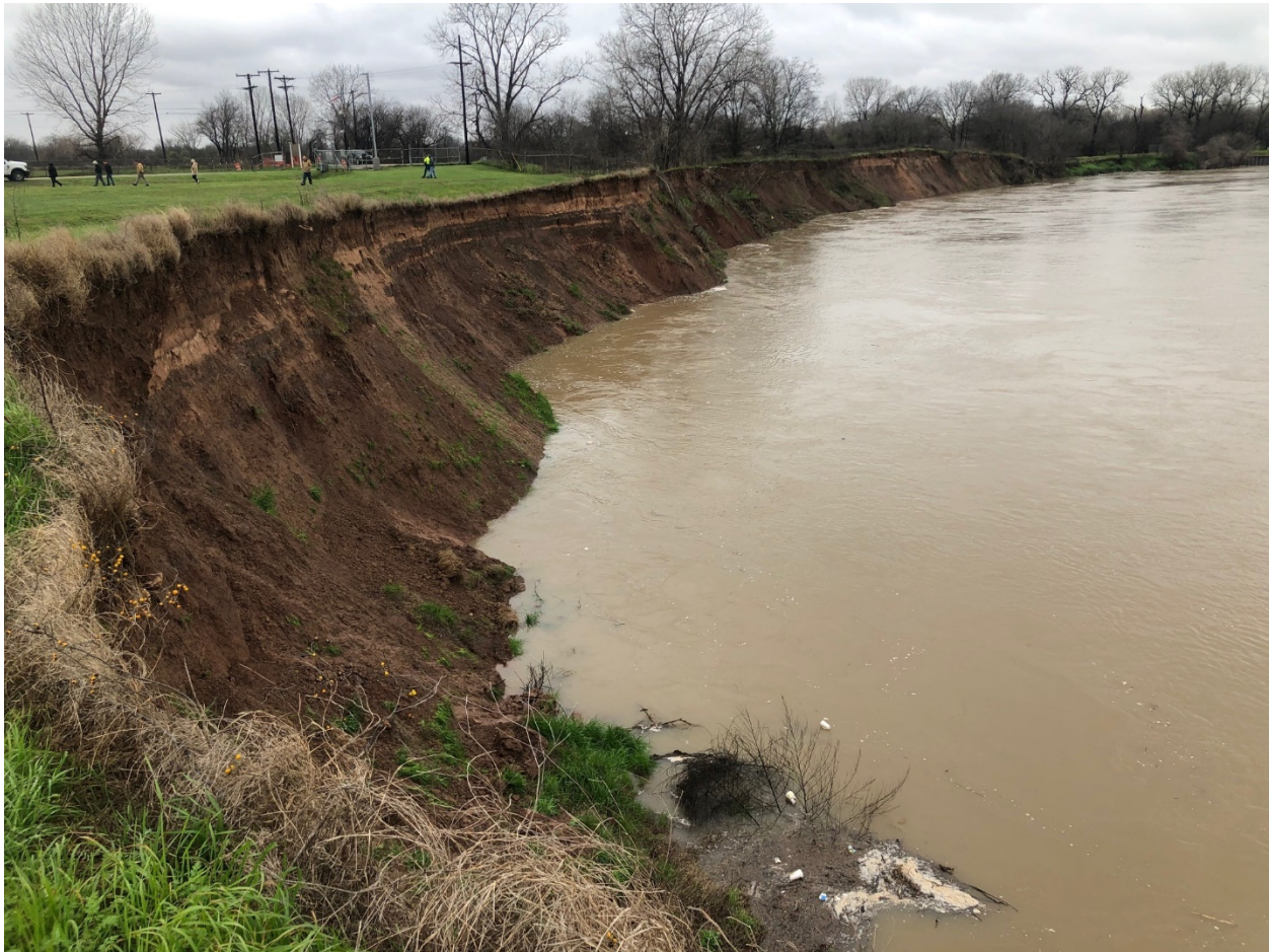
Looking upstream from the Waco Waste Water Treatment Plant, shows the embankment damage as of February 20, 2020.
