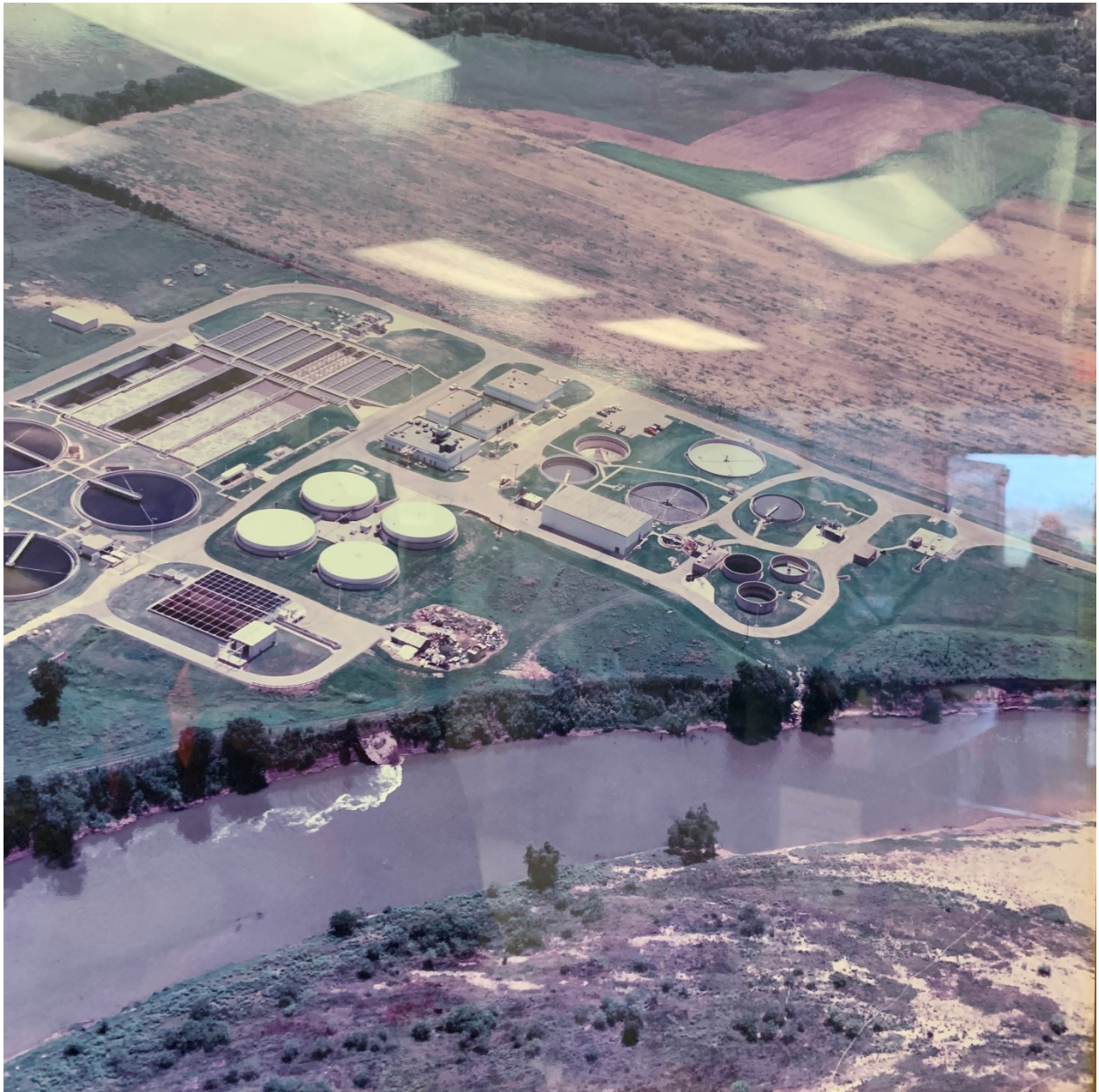
Waco Waste Water Treatment Plant Aerial taken in the early to mid-1990s.
